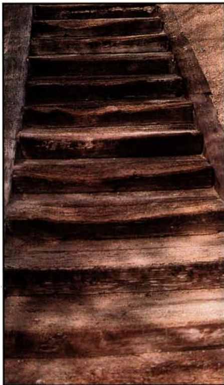
One drawback of spikeless golf shoes is the lack of traction on wood surfaces such as railroad tie steps and bridges. Various types of coverings can be used, such as rubber mats, to improve traction.
