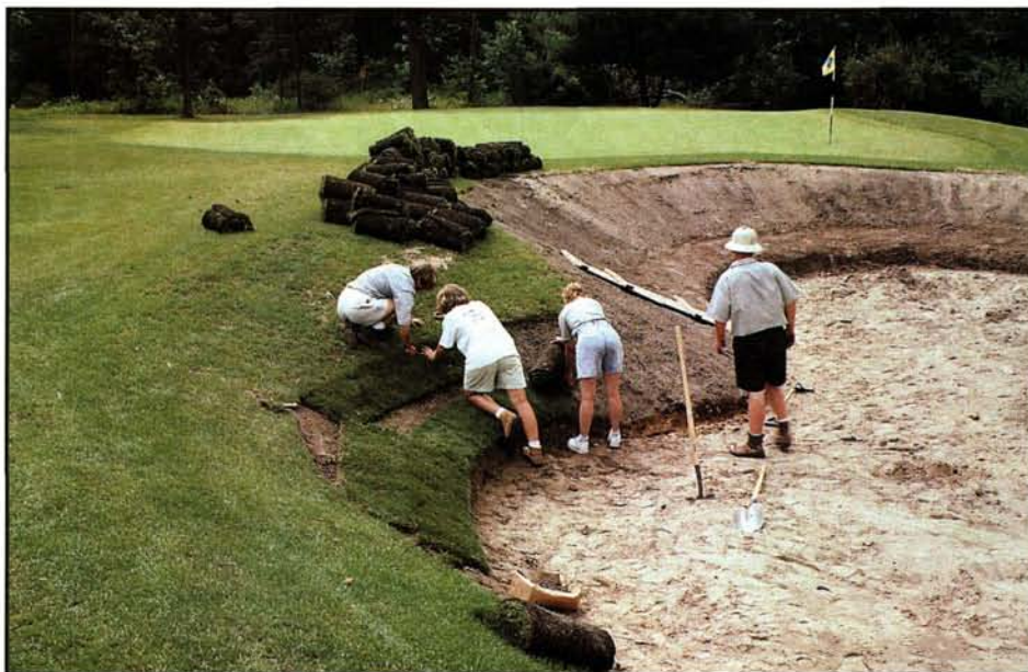
Be sure to include the turf adjacent to greenside bunkers whenever a surrounds renovation project is undertaken.
