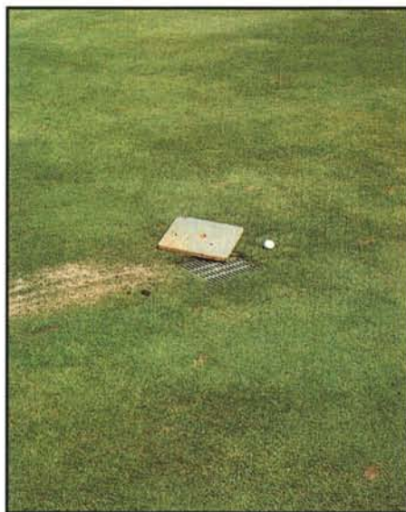
Temporary covers for drain inlets can be made from a variety of different materials. When installed prior to pesticide and fertilizer applications, they can help protect water quality.
