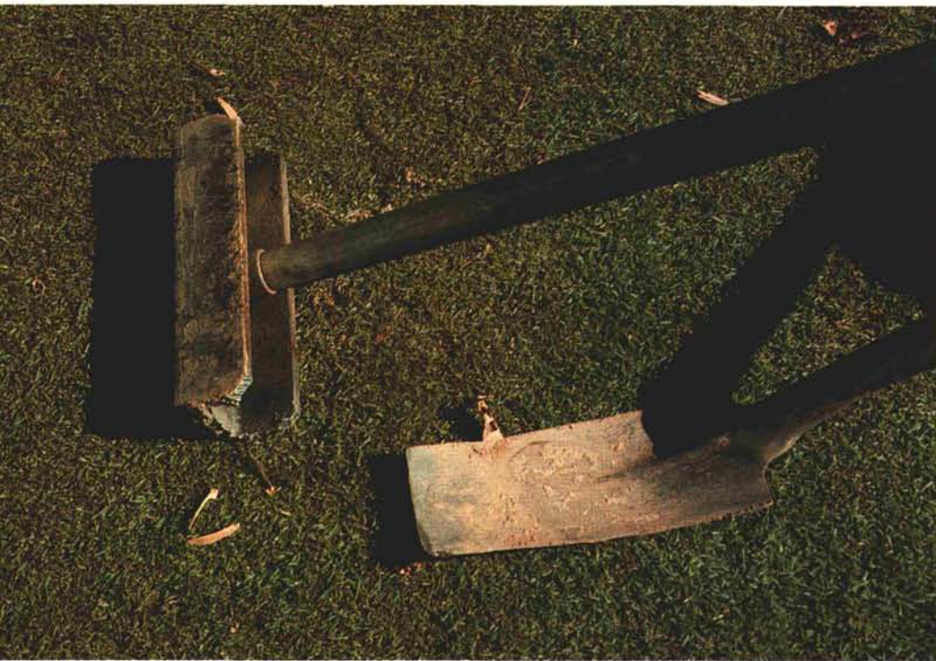
Essential tools included a narrow shovel and a tamping device made especially for the project.
