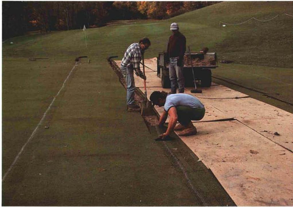
Great care was taken to replace the sod as it had been removed.
