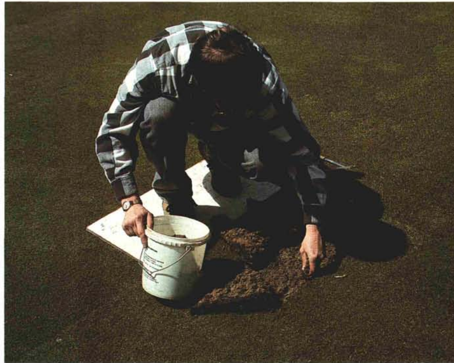
(Above left) The following spring, trench lines were topdressed several times to account for some slight settling.
