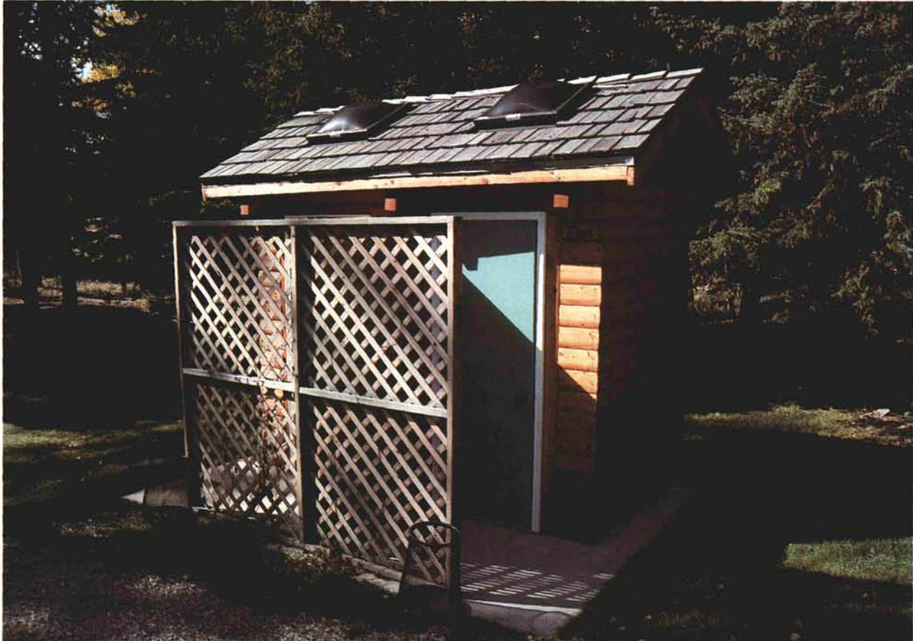
This well-designed, low-cost restroom facility gets its water supply from the irrigation system around a nearby green. The skylights provide adequate interior illumination.
