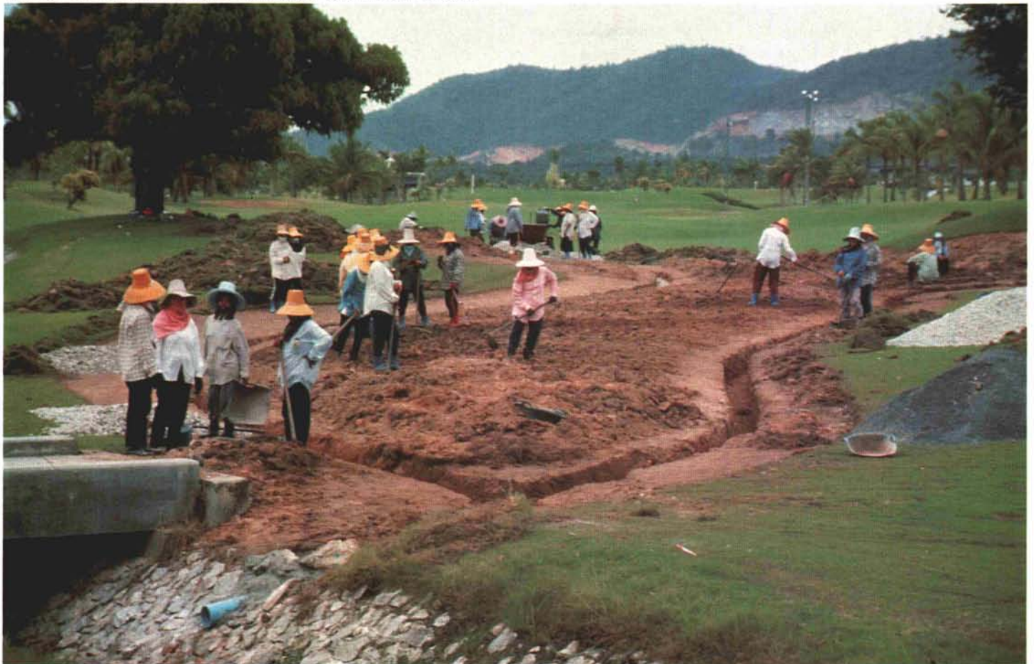
Drainage installation occurring 18 months after construction. Malaysia.
