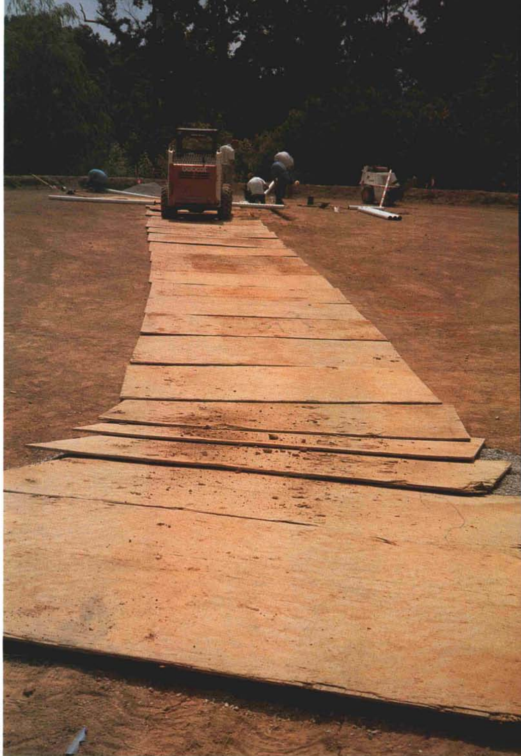
Plywood protects the subgrade surface so that the small skid loader can bring in the gravel and choker layer materials.
