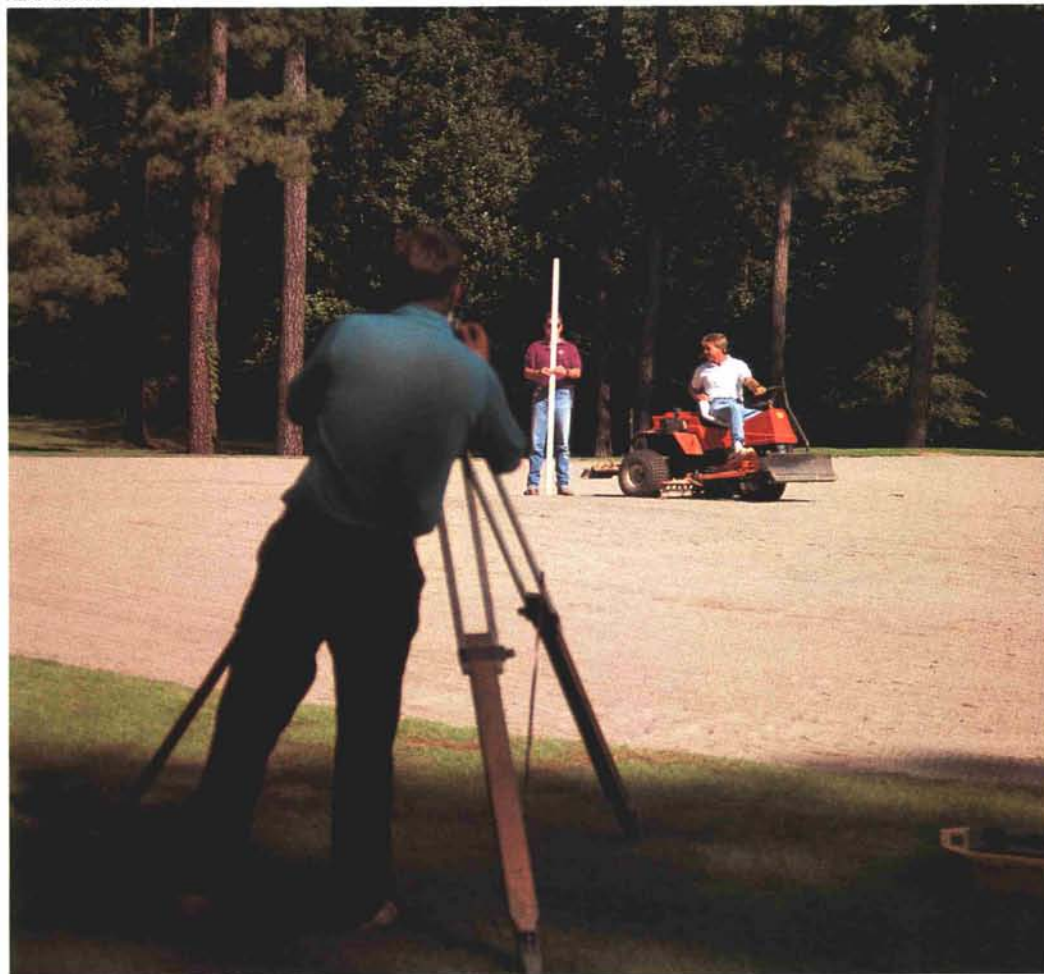
To insure that there are no pockets and that the green has positive surface drainage, a level and transit should be used in conjunction with a mechanical bunker rake.
