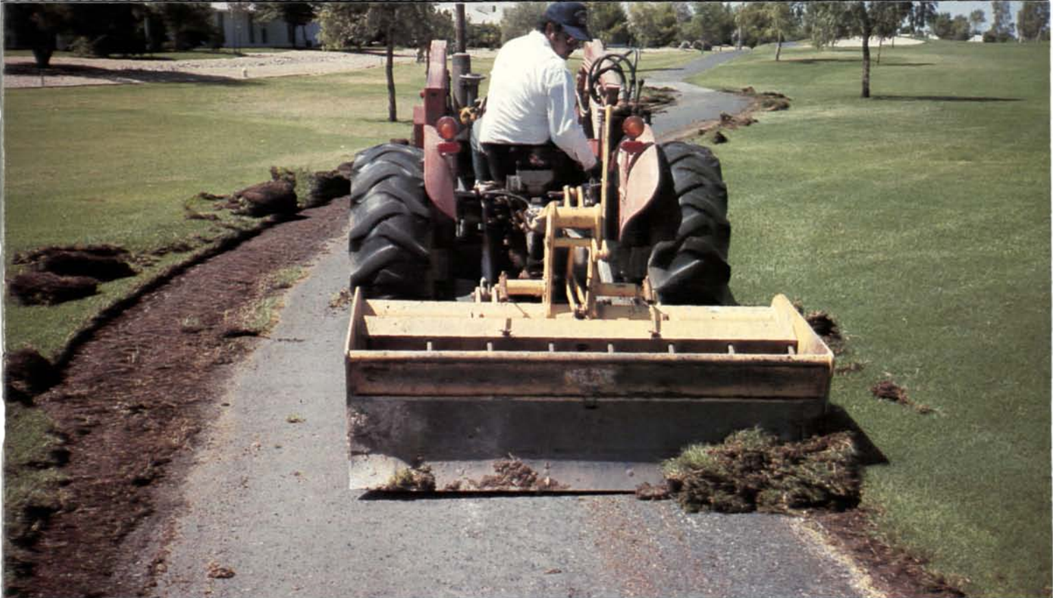
(Above) Ignoring the need to edge cart paths leads to premature asphalt deterioration and gives golfers the impression that the maintenance staff has little regard for good housekeeping.
