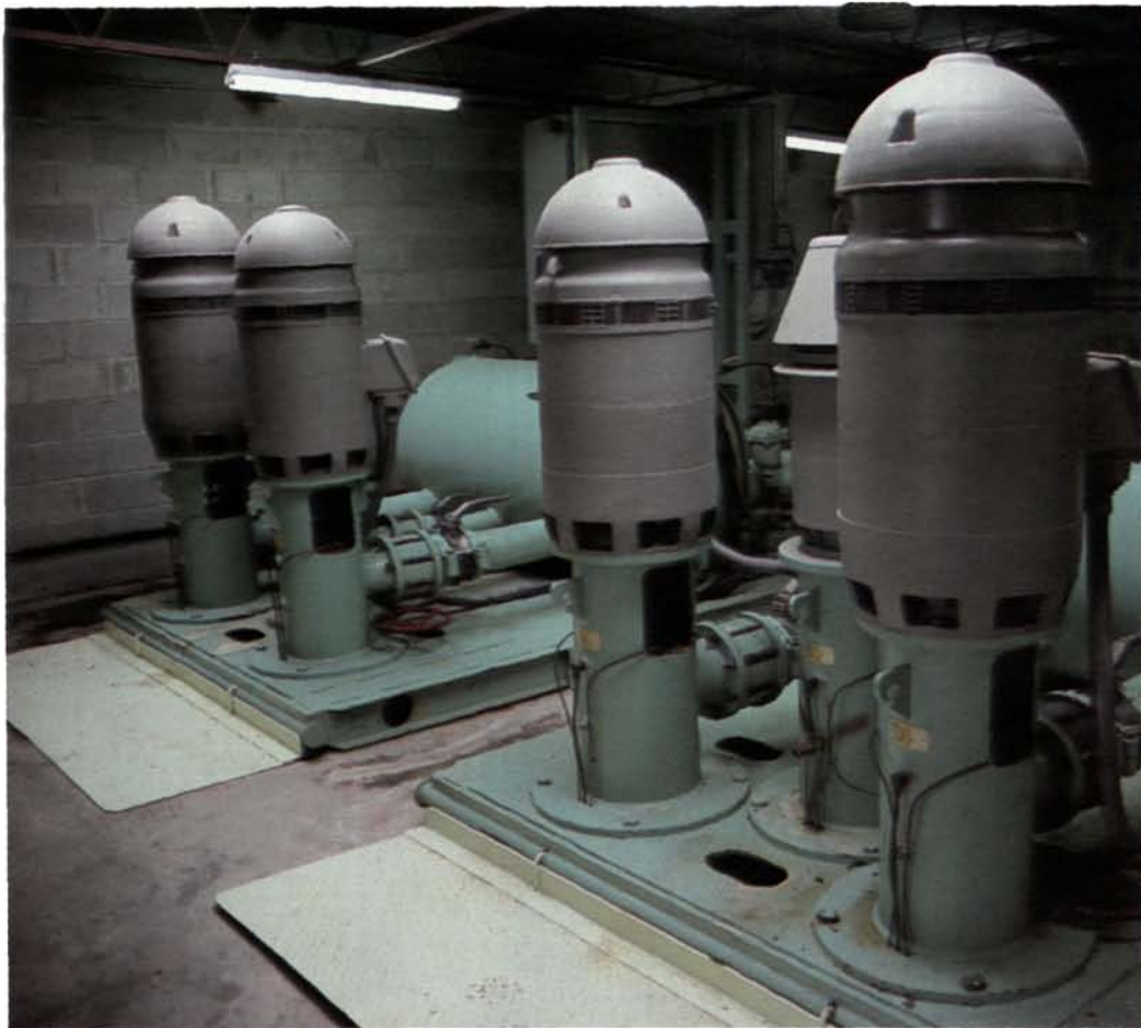
Understanding sophisticated irrigation systems is just one of the superintendent's responsibilities.
