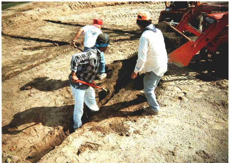
Into the trenches for drainage installation.
