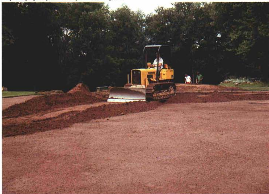
Preparing a firm foundation for a USGA green.
