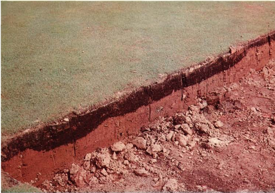
On-site mixing failed (Georgia, 1958)
