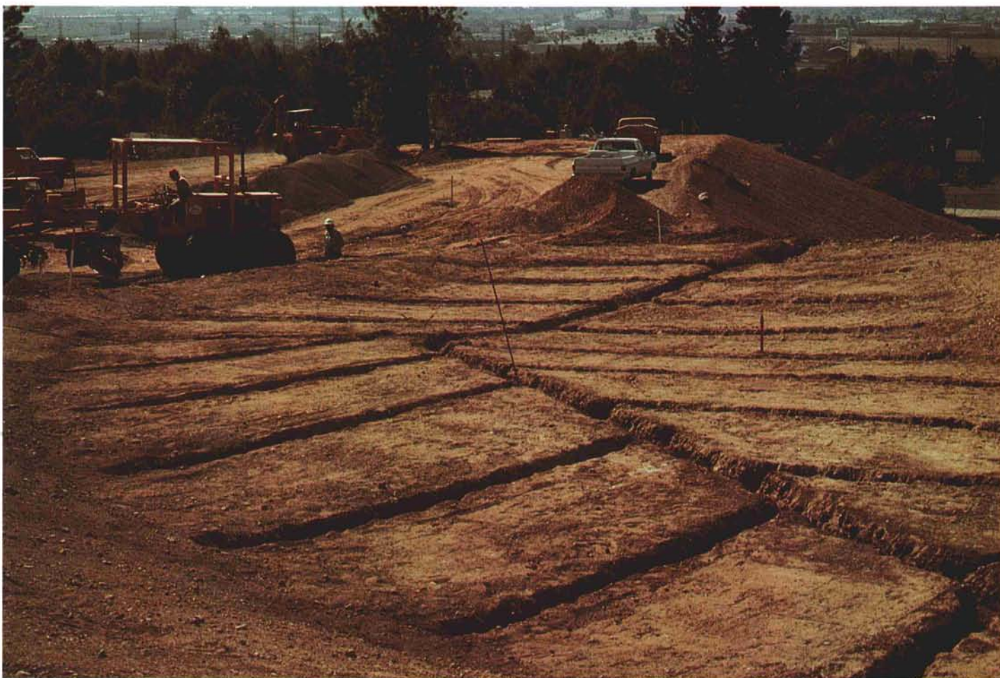
A properly built USGA green starts with good drainage.
