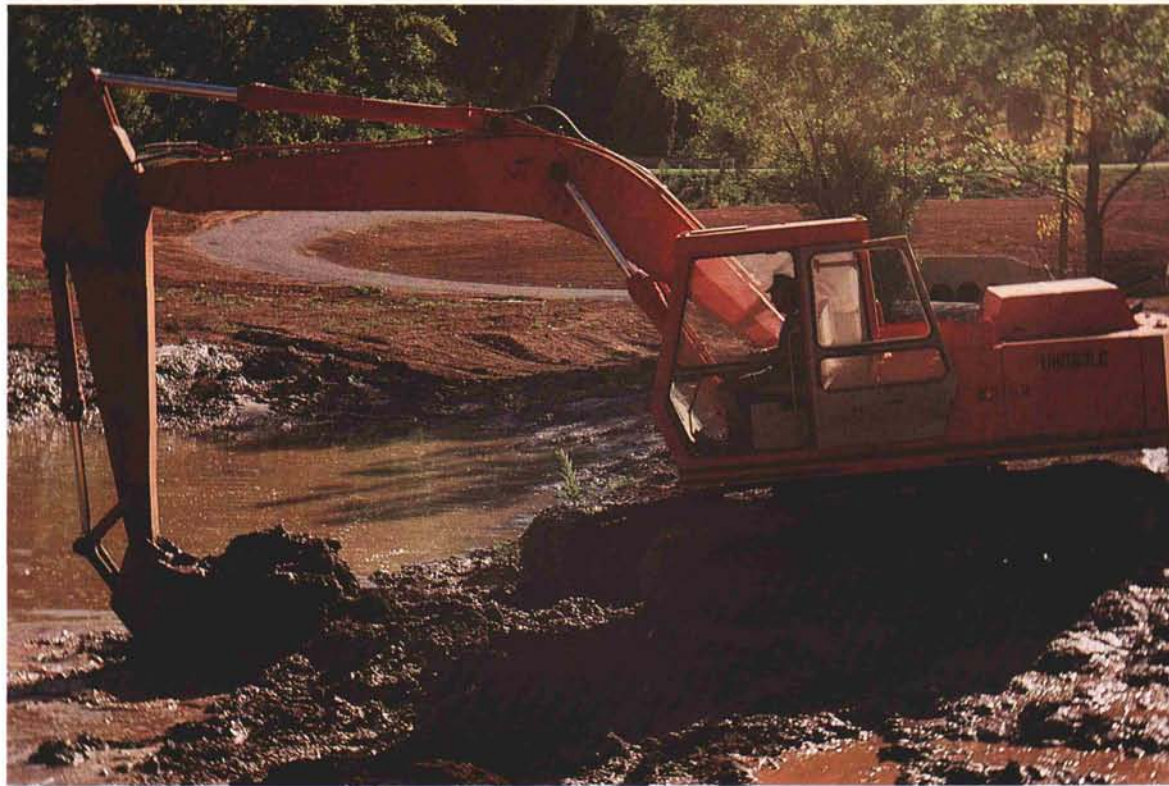
(Right) A track-hoe enlarging a lake into a water hazard.
