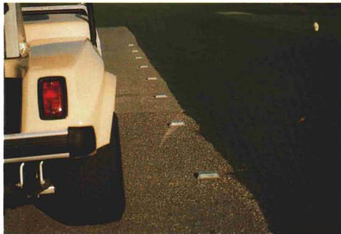
Reflectors placed at the edge of cart paths help prevent carts from damaging adjacent turf.
