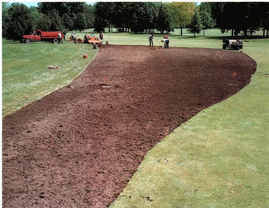
The old rough has been stripped and made ready for Kentucky bluegrass sod.
