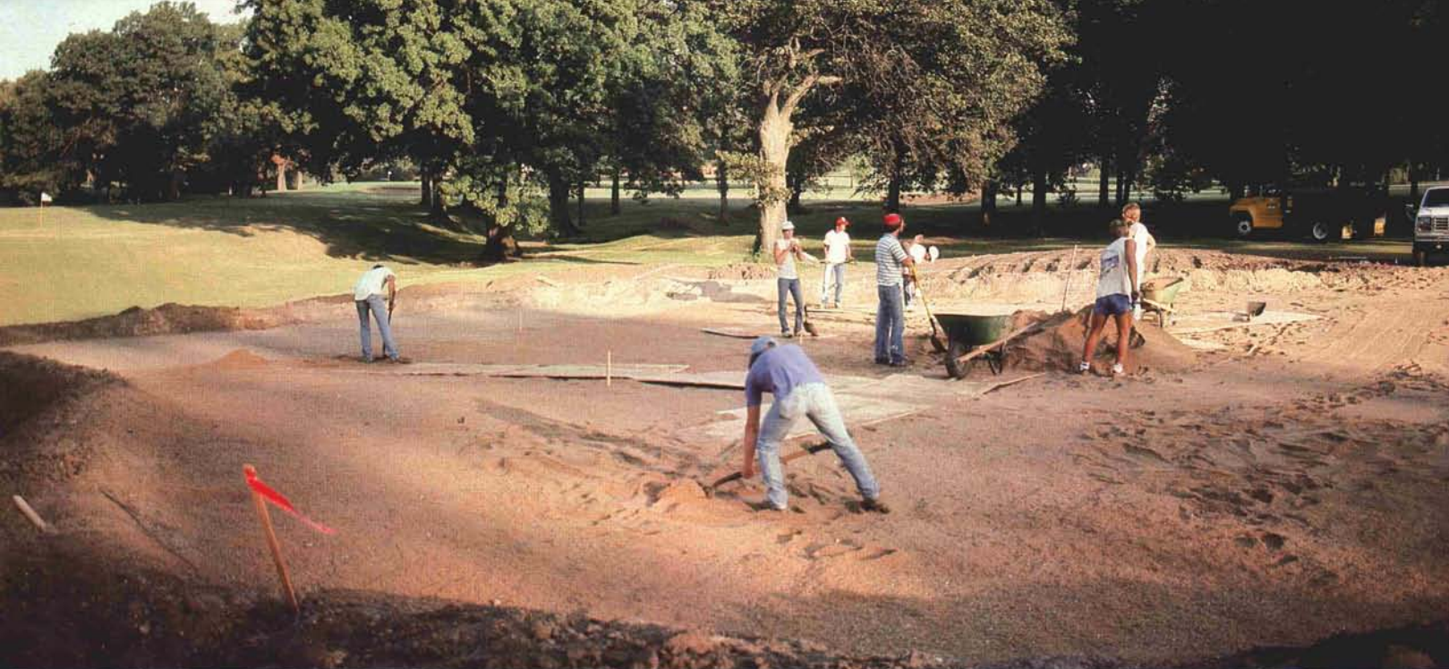
Spreading the 2" sand layer was easier and faster than expected.
