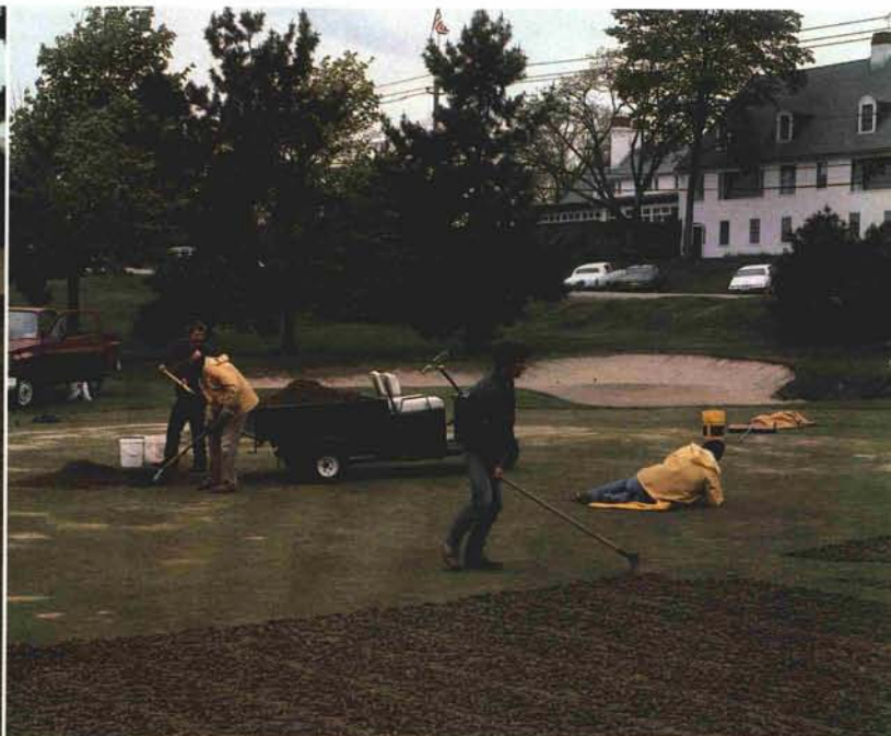
Removing the cores.
