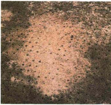
The damaged area.
