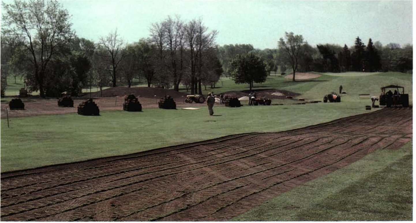
(Above) In May a sod harvester, operating in right background, cuts and palletizes square yard rolls of bentgrass sod to be moved to new location half a fairway away. Stripped area will be new rough.
