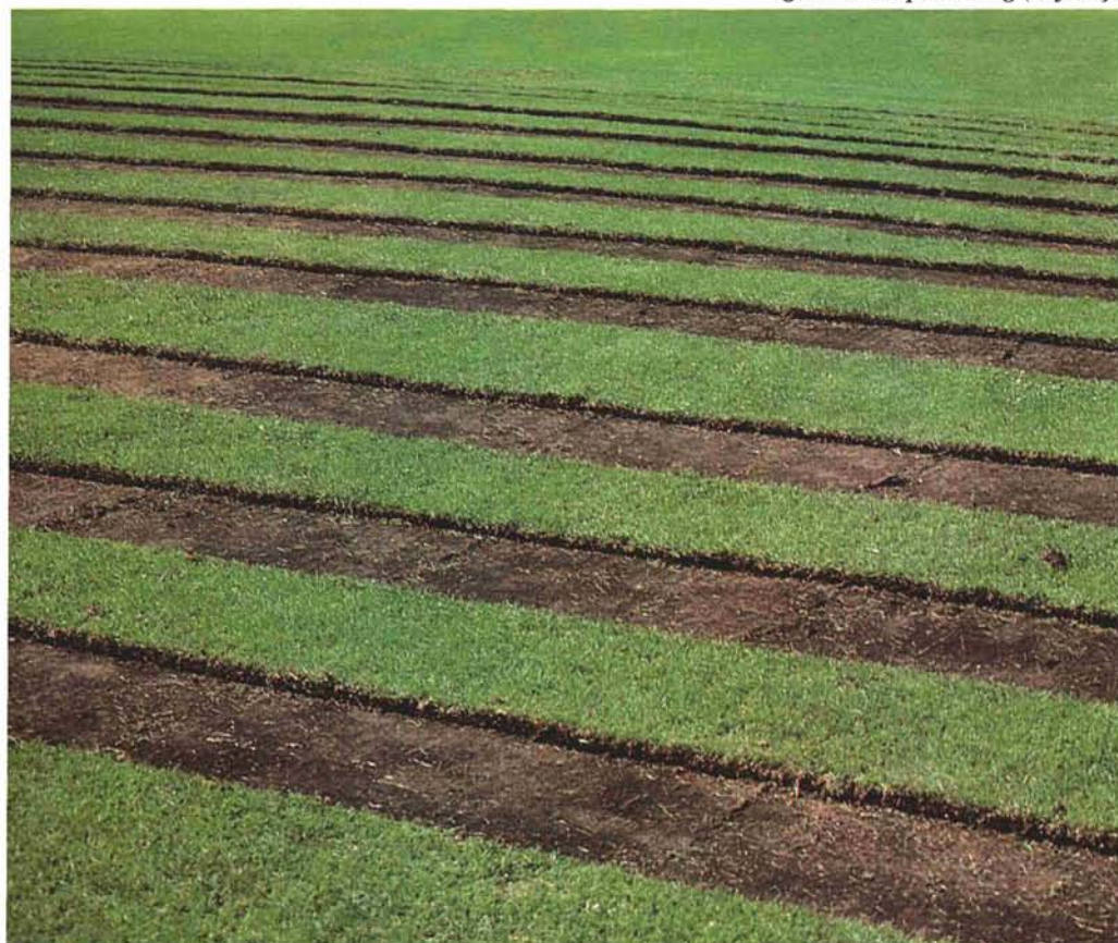
Figure 4. Strip sodding (before).
