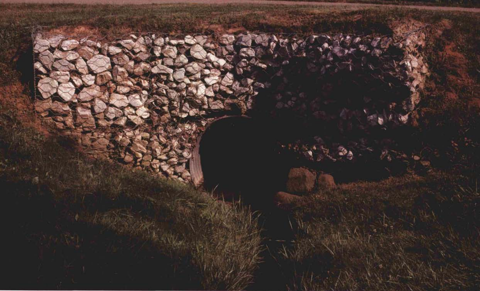
Gabions being used as a headwall.
