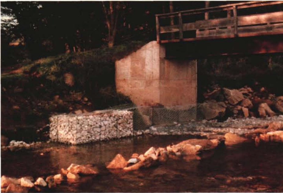
First gabions on the upper course (summer).
