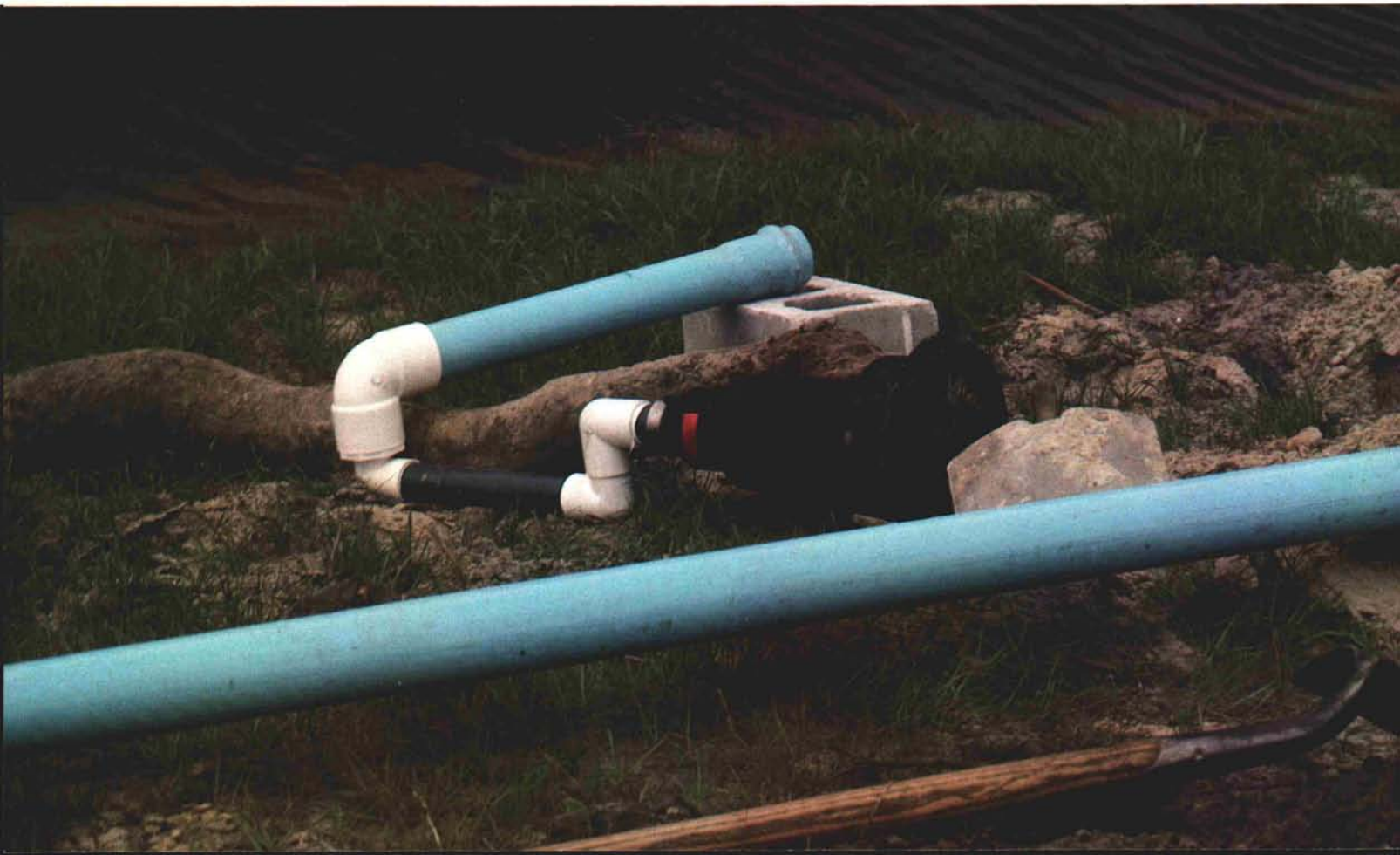
Swing joints of all PVC construction act as shock absorbers for the piping system. This one is ready to install.
