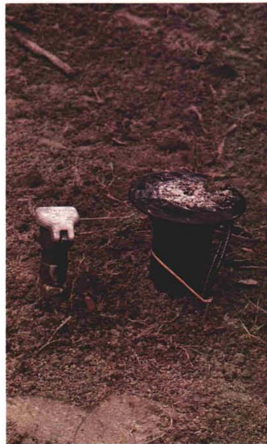
Quick couplers should be readily accessible and easy to locate.
