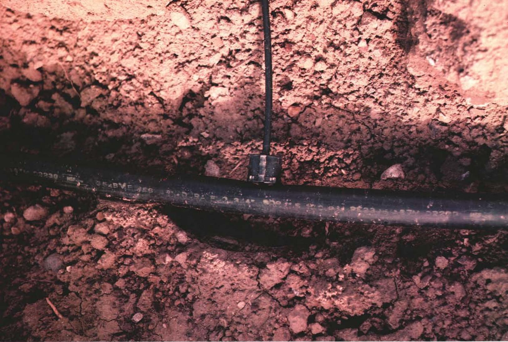
*Polyethylene tubing, emitter and "spaghetti" tubing in trench before burying.*
