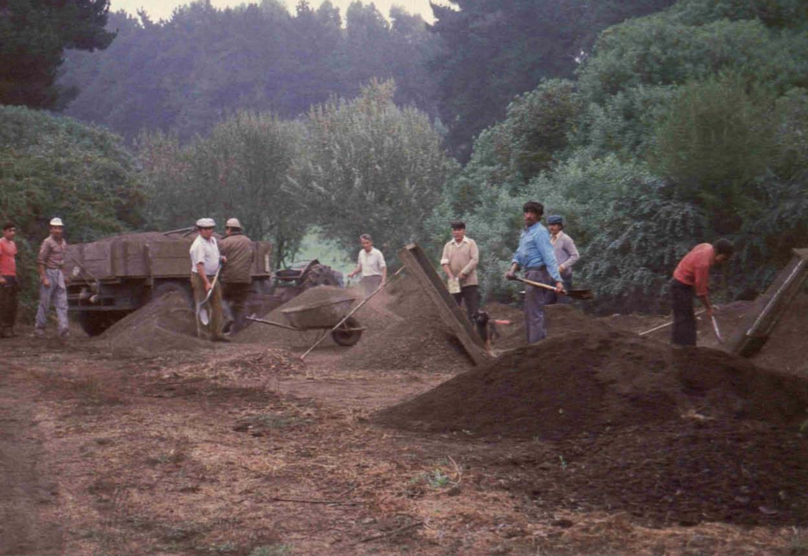
Mixing topsoil without modern equipment requires the entire work force.
