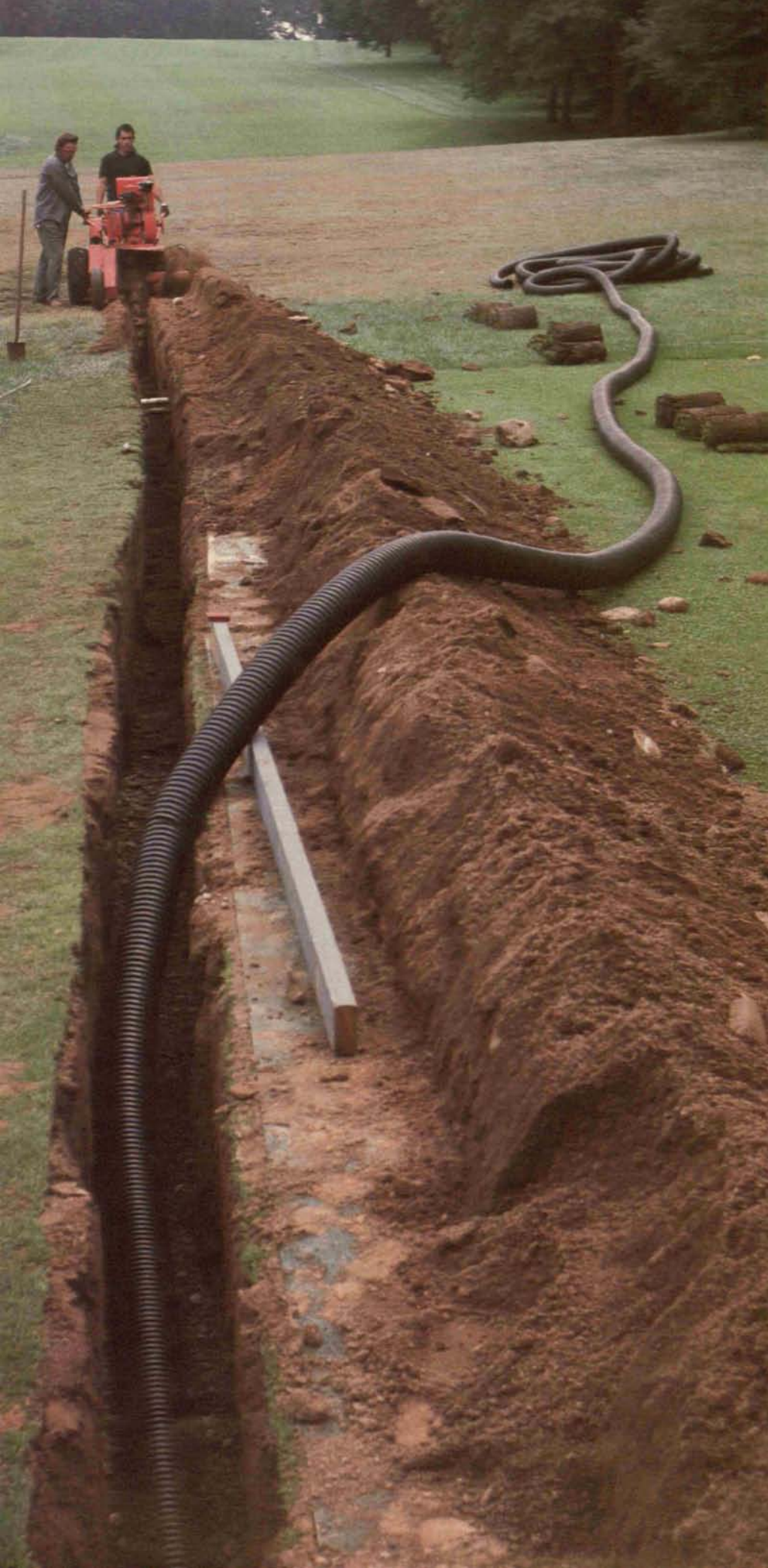
Figure 1. While the procedure is the same for every drain line, the difference in an open stone trench is that the soil is hauled away and the pipe is completely covered with gravel or crushed stone. Ridgewood Country Club, New Jersey.
