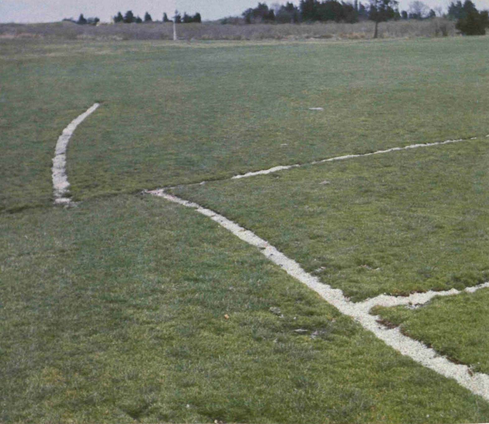
Figure 2. Pattern showing versatility of a slit trench system — two lines in gridiron fashion empty into a line that carries the excess water down natural incline. Note crushed stone in trench is filled to turf level. Wildwood Country Club, New Jersey.
