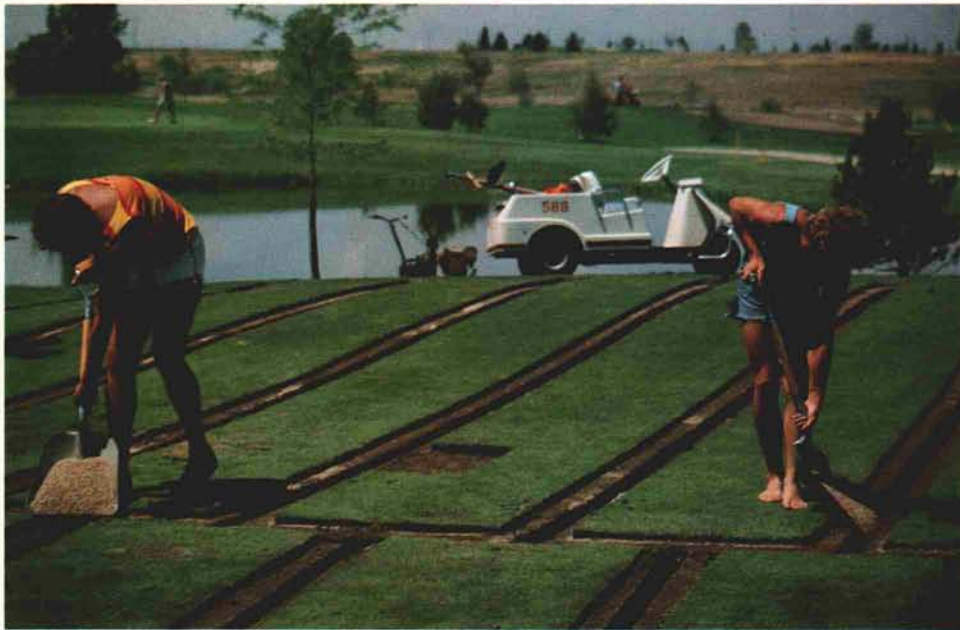
(Top, left) Lateral drain trenching and clean-up.
