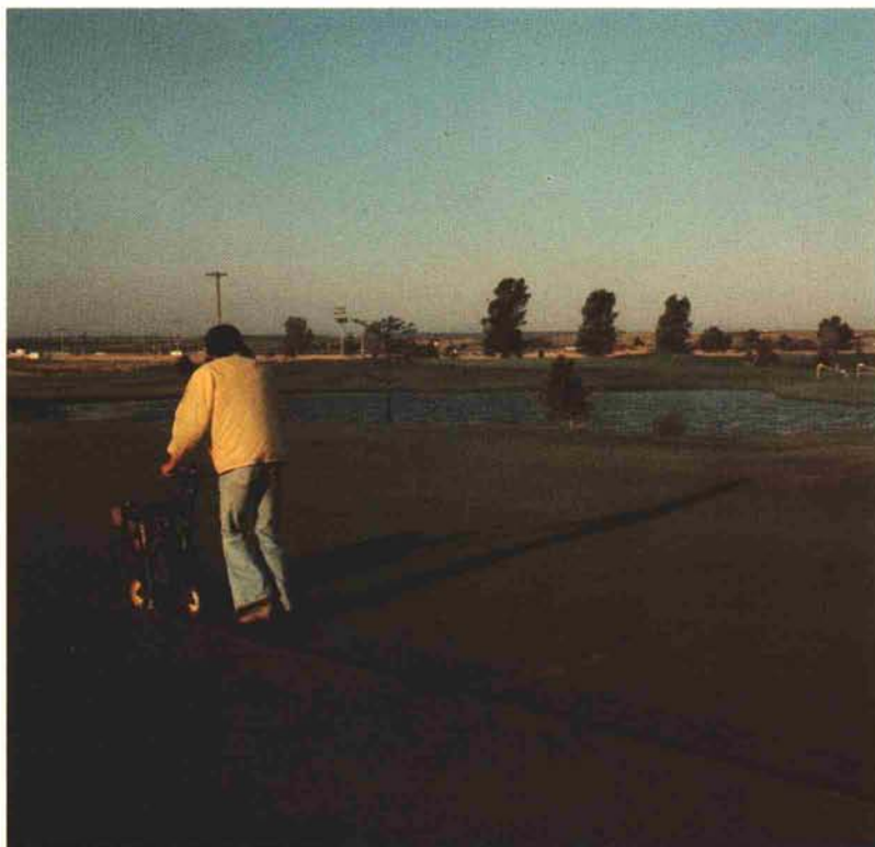
(Left) Sod is stripped where main drain is to be installed.
