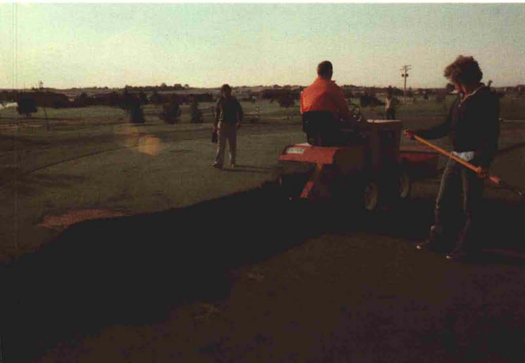
(Left) Trenching for the main line.
