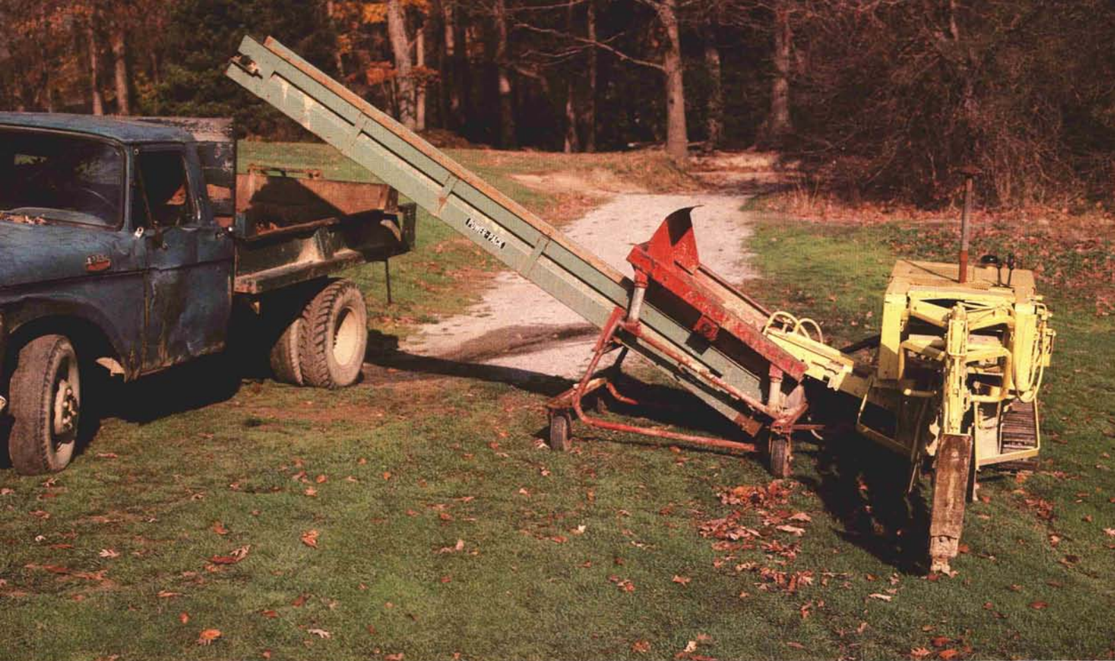
Equipment used to remove soil from ditching site.
