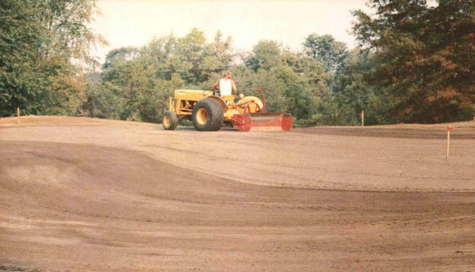
Making the final grade with the grader box prior to overseeding the green.
