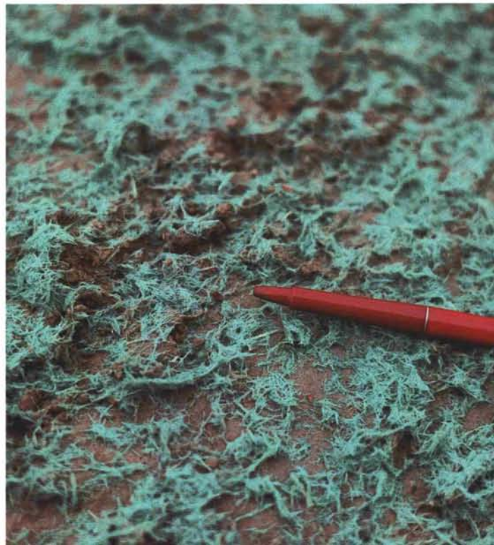
Fiber cover after hydroseeding. Pen points to actual seeds.
