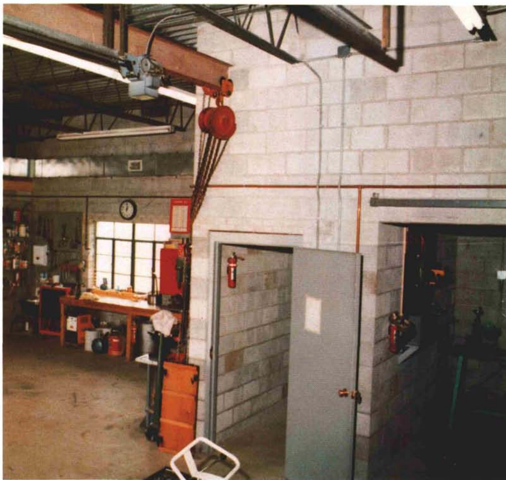
(Above) View of maintenance shop's new interior.
