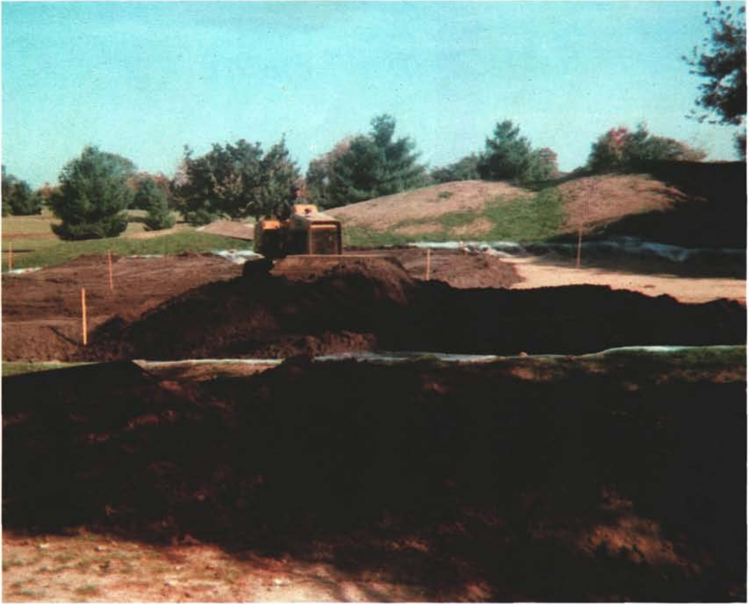
Spreading a prepared topmix for a green rebuilt to USGA Green Section specifications.
