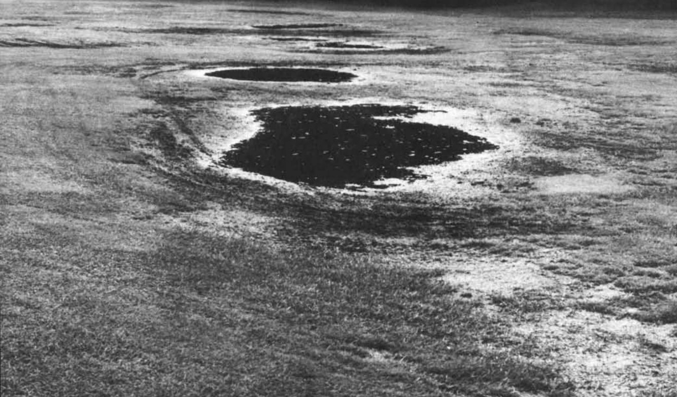
Fundamental problems must be corrected before renovation is undertaken.
