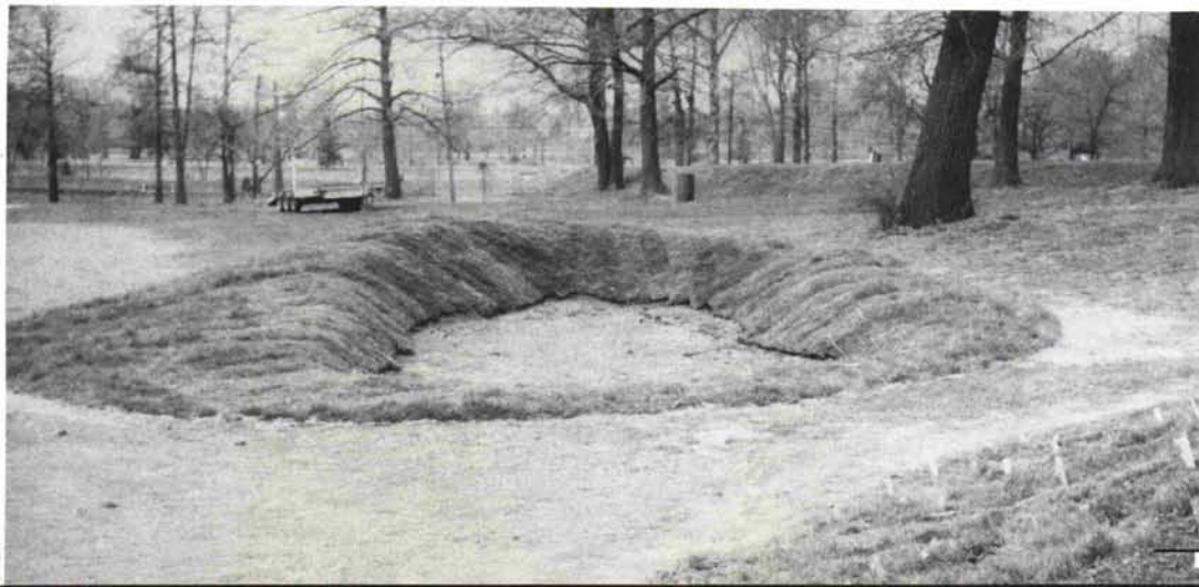
Figure 1. Old style sand bunkers under construction.
