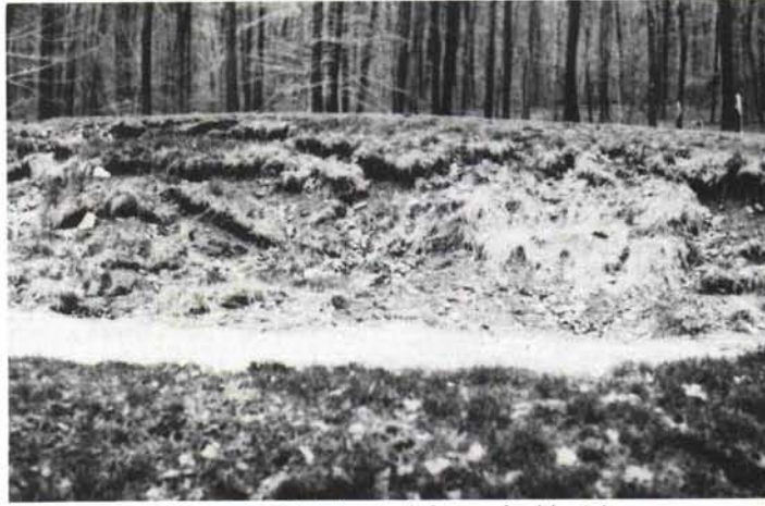
Figure 2. Deteriorated face of old style bunker, a problem on many golf courses.
