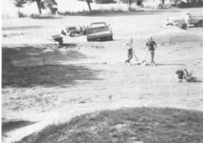
Stripping old green and removing soil to desired sub-grade.
