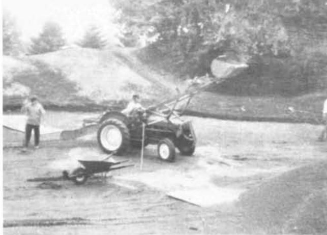
Pea gravel over drain lines and sub-grade to form stone base.
