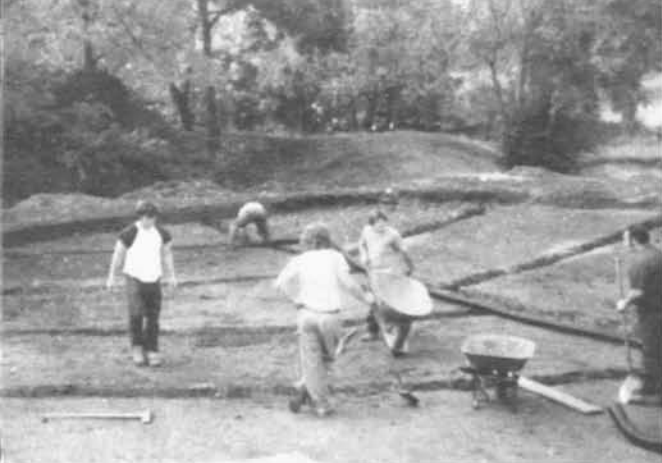
Installing drain lines in the sub-grade.
