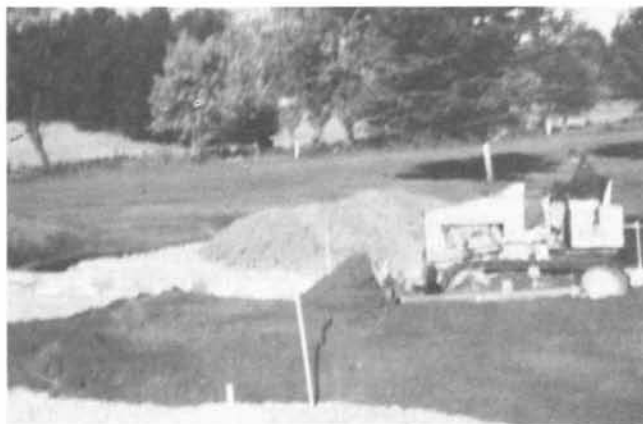
Top soil spreading operation.
