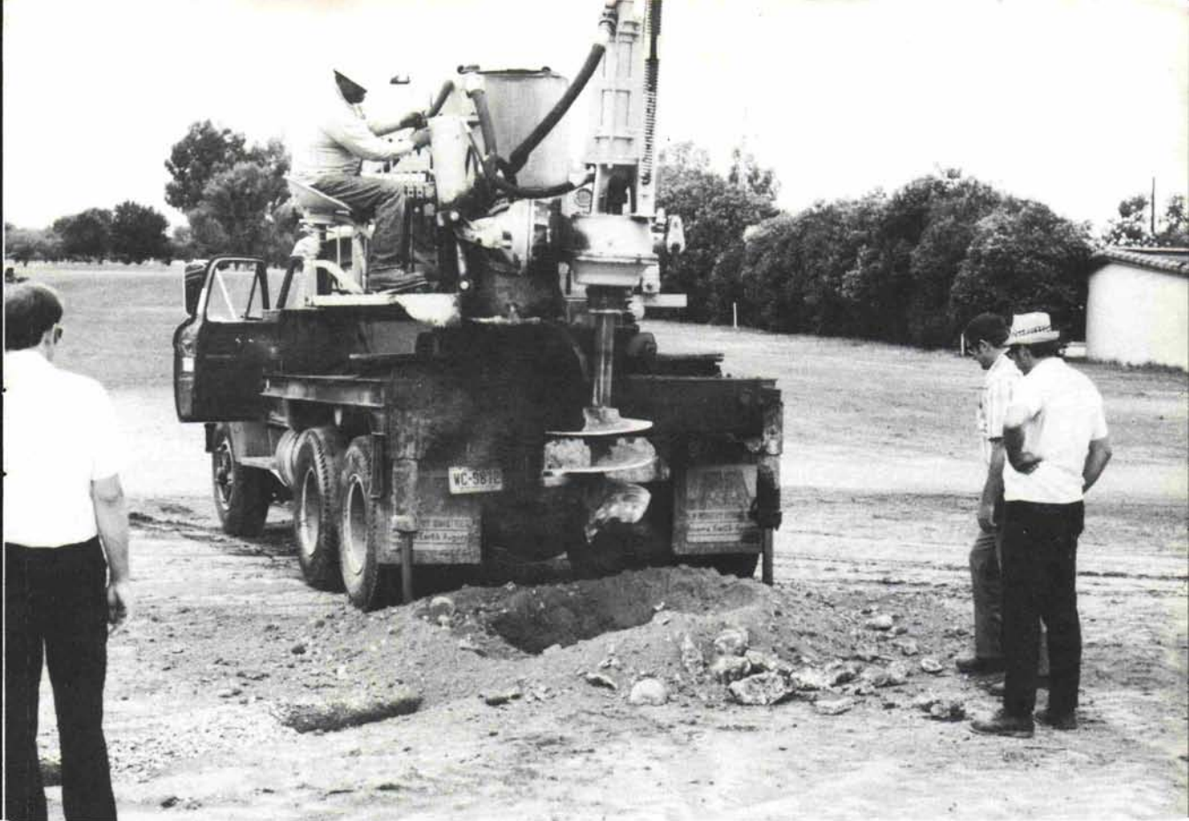
Deep dry wells may be needed for drain points for tile lines.
