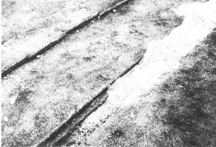
Coarse sand tops off the trench.
