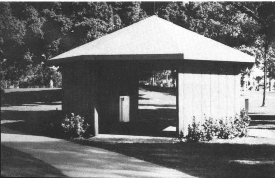
The finished product; landscaping, water cooler and all.
