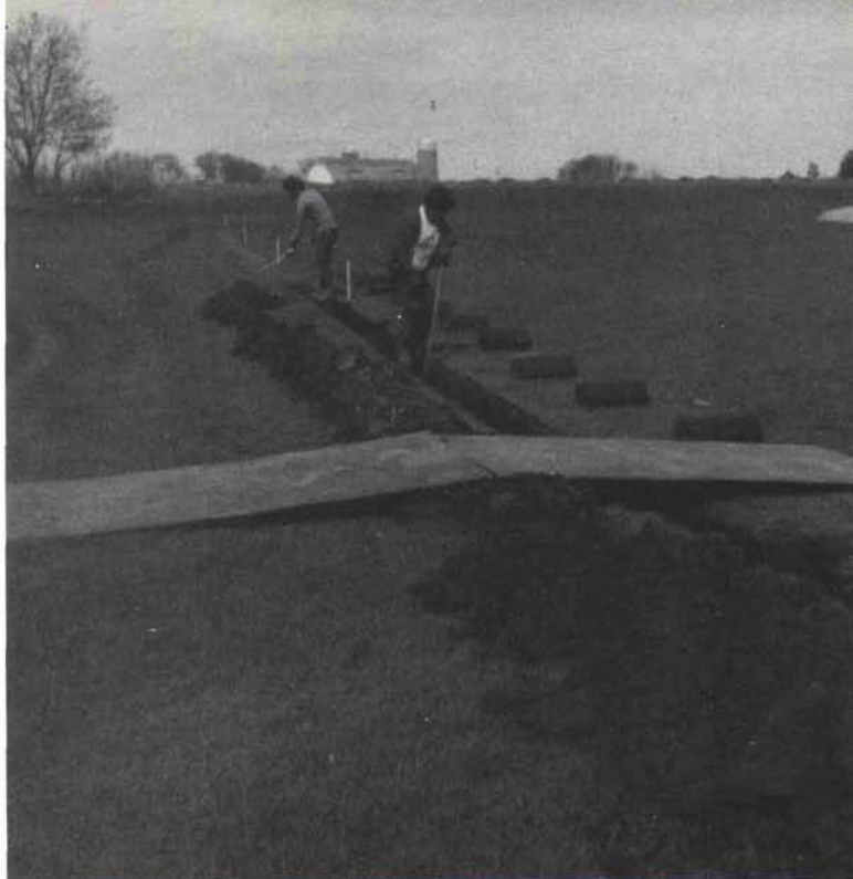
Removing the sod, digging the trench; the pieces of plywood allow golf cars to cross.
