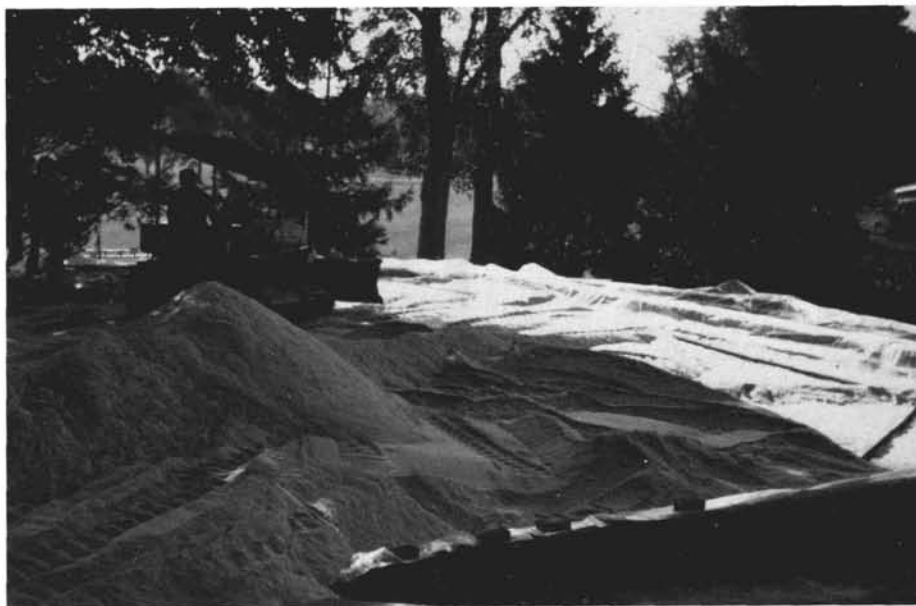
Sand being graded over polyethylene liner and drainage pipe.
