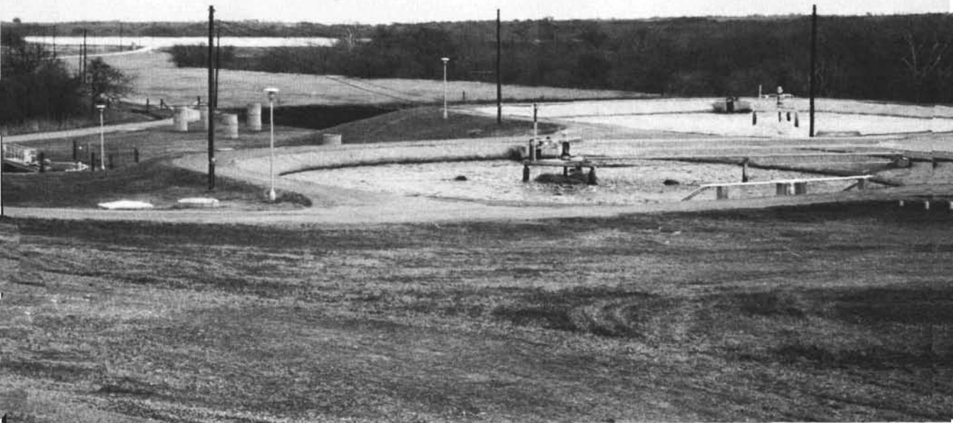
Several million gallons per day sewage plant at Austin, Texas with a 40-acre lake in left background. New golf course will be entirely irrigated by effluent water from this plant.
