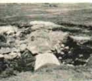
Sand bunker drainage is important.
