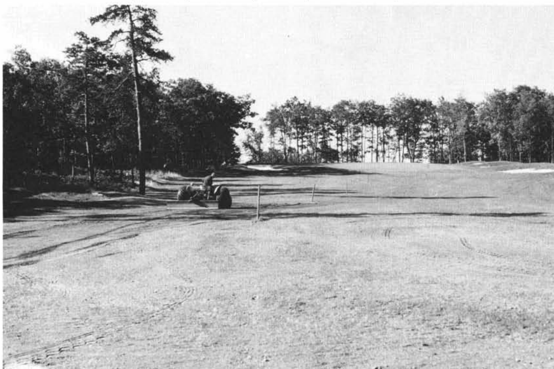
Top dressing and leveling a fairway as it nears completion.
