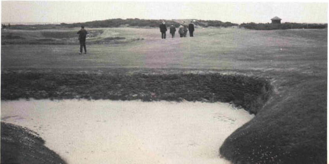
A fairway bunker at St. Andrews, Scotland showing the shoring up of the sides.
