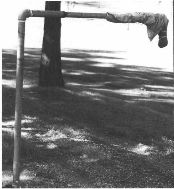
Supt. Roy Mackintosh, Twin Hills C.C., Longmeadow, Mass., set up this permanent installation for filling the spray rig efficiently.
