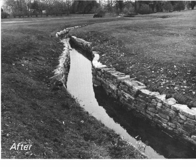
of the wall crumbled and erosion was once again a problem on the stream banks. It was decided most practical to rebuild the wall completely. Because it seemed more economical to use our own labor rather than hire an outside contractor, work on the wall was necessarily delayed until the latter part of August, 1970, when some labor time was available.
