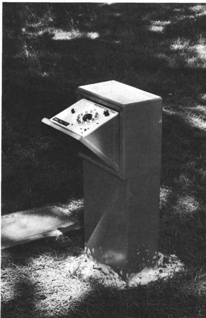
Pedestal mount controller for an underground irrigation sprinkling system.
