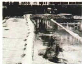
COVER PHOTO: The terrace was flooded to check for leaks in one step of building a Purr-Wick putting green.
