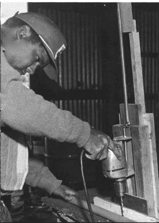
Superintendent Jack Jagur perforating the 1-inch plastic lateral lines.
