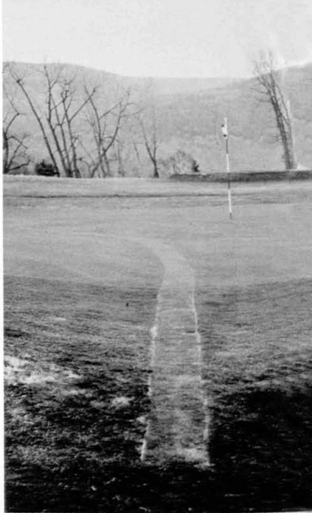
A sod cutter is used for aiding surface drainage on greens.
