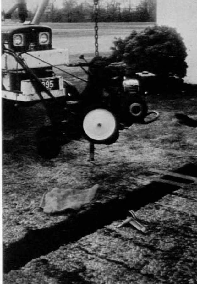
Sod cutter with mole attachment is used to install heating cables.
