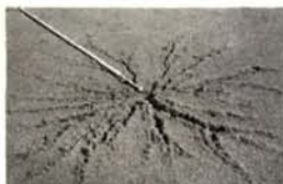
COVER PHOTO: A bolt of lightning struck the metal hole liner on this green and caused extensive damage to the turf.
