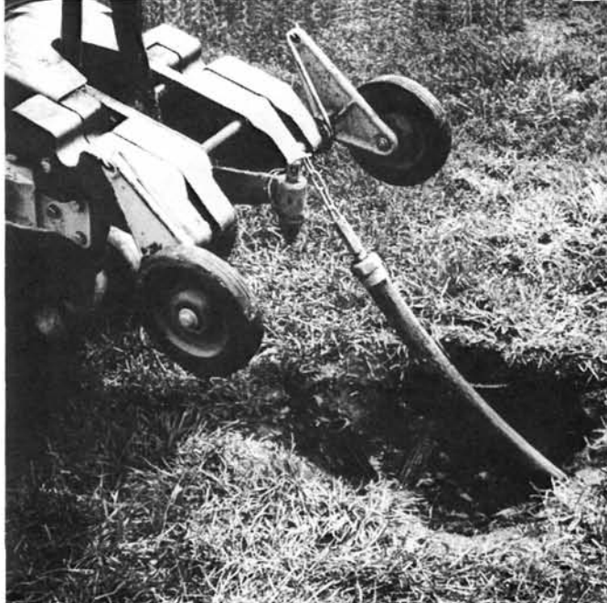
Figure V, mole method of laying pipe.
