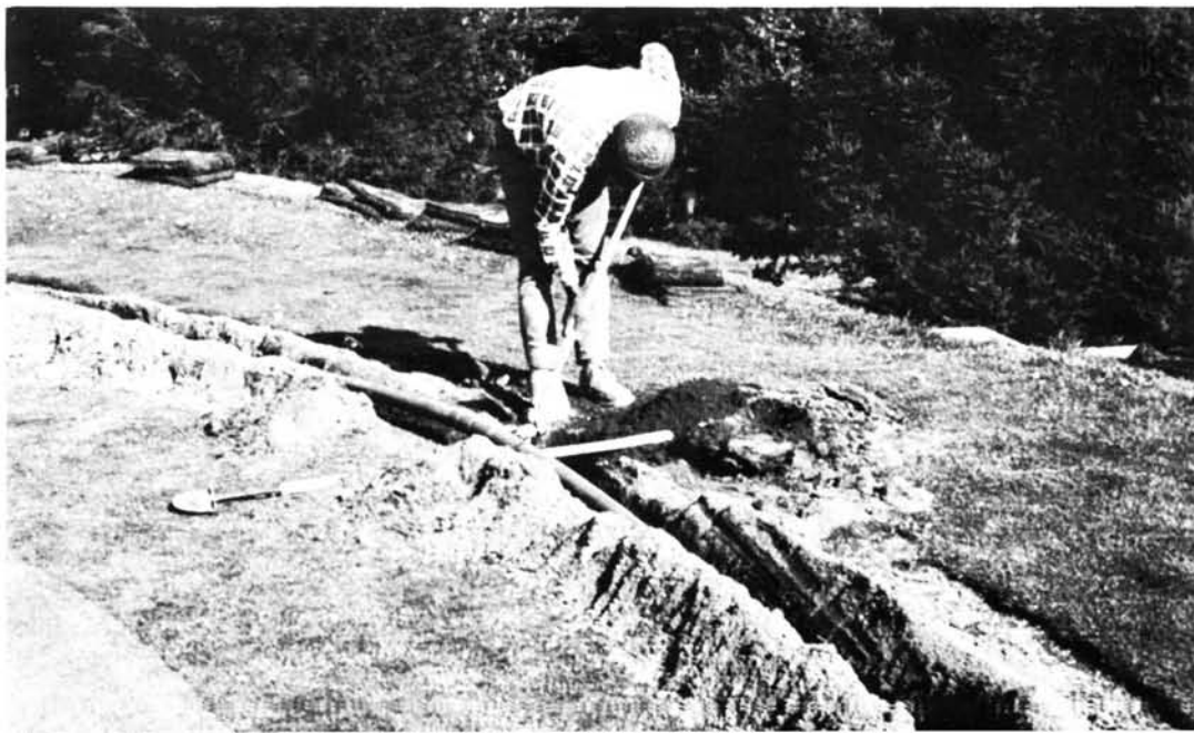
Figure IV, trenching method of laying pipe.
